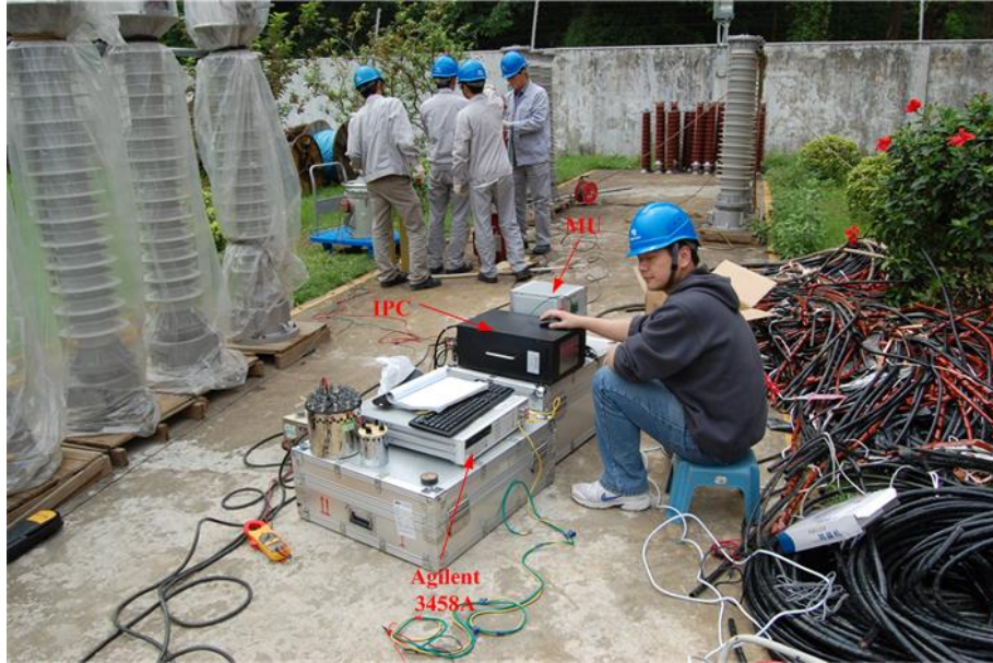
Fig. 11. The picture of on-site calibration in Sanxiang substation.
